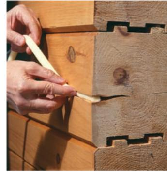
1. Install backer rod into a clean, stained check to the appropriate depth. (See Fundamental Application Guidelines.)
