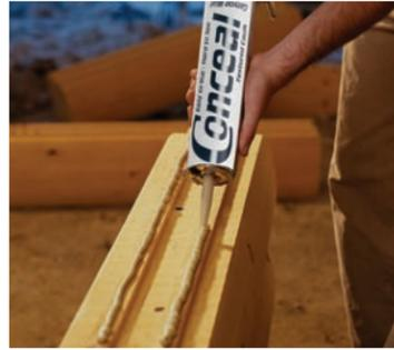
Apply a bead(s) according to the log home manufacturer's instructions. Stack the next log and repeat. Don't allow caulk to skin over prior to stacking.
