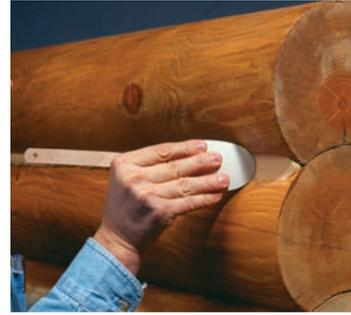
2. Tool to ensure a tight seal to the top and bottom of the caulk line leaving at least 1/4" depth of caulk in the center of the joint.\*
